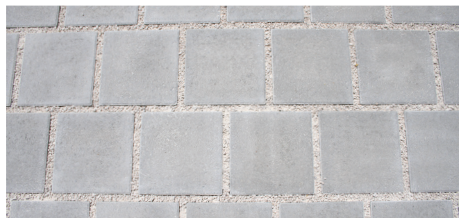
Pose joints croisés = CIRCULABLE T3-4
