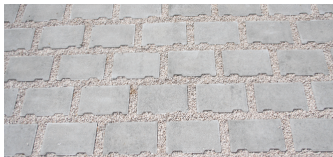
Pose joints croisés = CIRCULABLE T3-4
